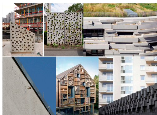
Figure 1. Upper row left to bottom right: concrete building envelope with integrated planters Chartier-Dalix Architects (source: Chartier-Dalix Architects Photo credit: Takuji Shimmura). Lower row left to right: Animal-Aided Design building integrated bird nest in the Brantstraße in Munich (source: Animal Aided Design). Mellor Primary School habitat wall by Sarah Wigglesworth architects (source: Lower row left to right: Animal wall (bats)—art installation in Cardiff bay by Gitta Gschwendtner (Source: Gitta Gschwendtner. Photo credit: Kiran Ridley).
